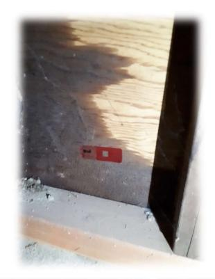
Wet wood by a pipe going through the building envelope in the west wing crawlspace. Sample B06 contained ascospore, basidiospores, hyphal fragment, and Stachybotrys/Memnoniella spores.
