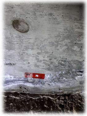
Water stained fungal growth along the concrete wall of the crawlspace next to (and south of) the exposed plywood of the building envelope in the west wing.
