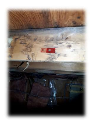
Water stained wood in the ceiling space above the central section of the school. Sample B04 contained ascospore, basidiospores, *Cladosporium* spores, and myxomycetes spores.
