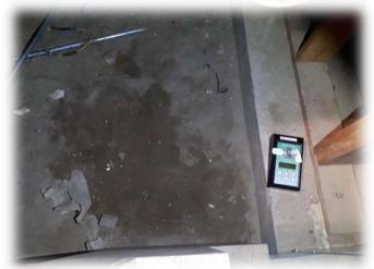
Damp dirt in the crawlspace under the stockroom after the water boiler was removed. Odour resembling *Penicillium* was detected from the damp dirt.
